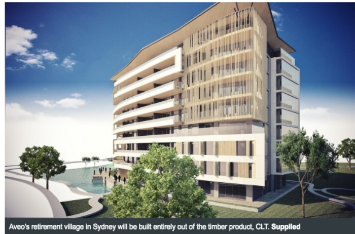
Aveo's retirement village in Sydney will be built entirely out of the timber product, CLT. Supplied
